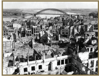
Bridge over the Rhine, Nijmegen. Courtesy of Everett Collection/Alamy.
